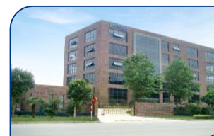
FUCA HVAC Automation
